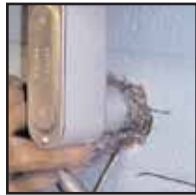
Around utility conduit.
