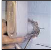
Around utility conduit.
