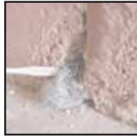
Exterior crack sealed.
